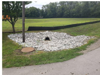
Rebuilt culverts around district
