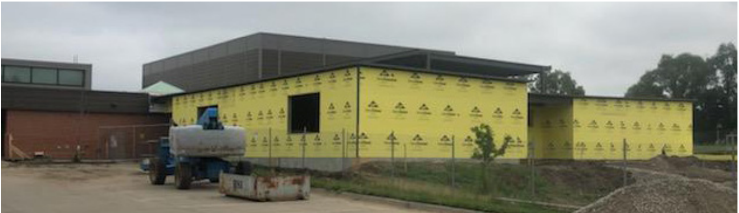
Cornell Elementary School third grade addition.
