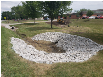
Rebuilt culverts around district
